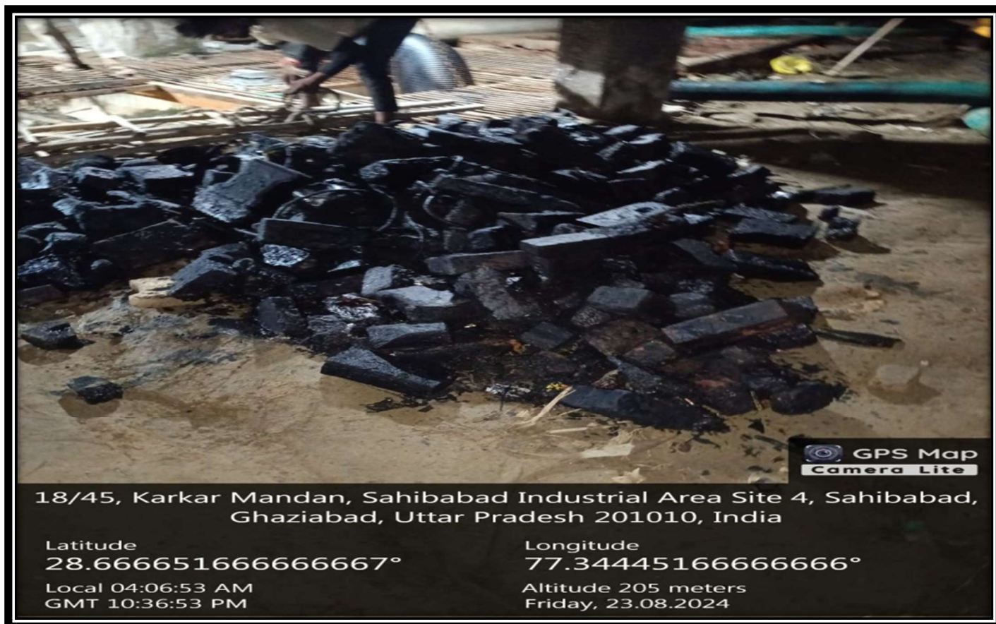
Tiles and bricks removed from well
