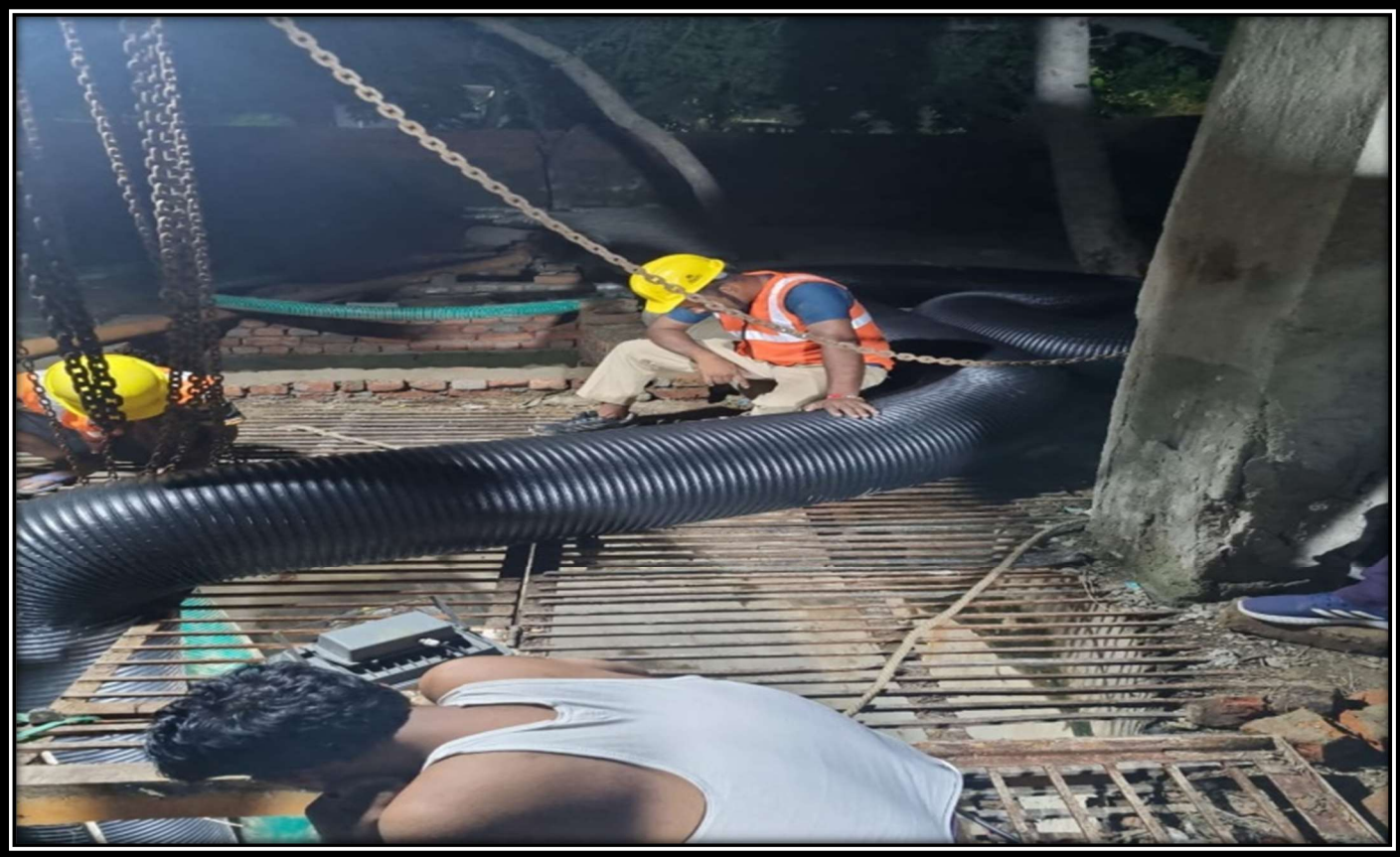
Installation of blower for removal of gases
