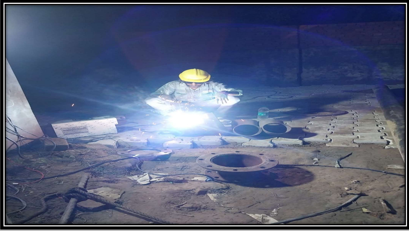
Fabrication work for installation of pumping plant
